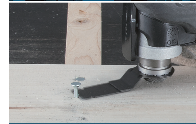
Flush cutting of nails
