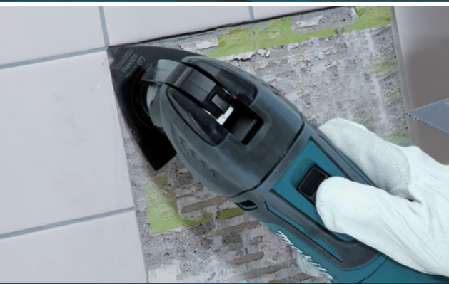
Removing mortar, tile adhesive
