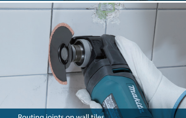
Routing joints on wall tiles
